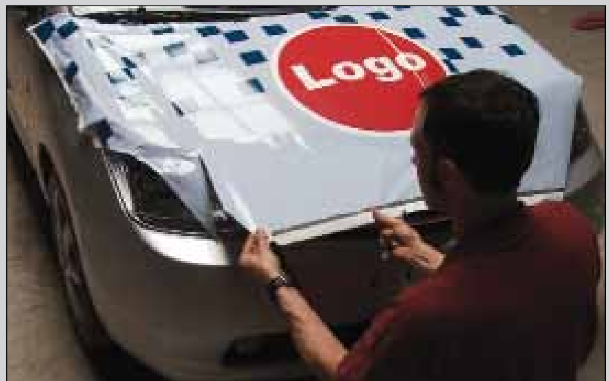
So many vehicles look good from a distance, but upon close inspection, they are peeling or lifting, particularly on bumpers, fenders and recessed areas. In most cases, this is simply due to the fact that the film was overstretched.
