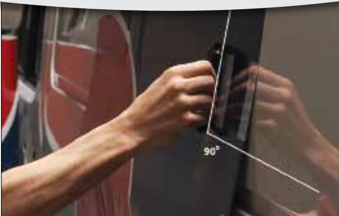
Squeegeeing at a 90-degree angle is too wide. Use too wide an angle and the film will bunch up at the bottom, which will lead to wrinkles, lower quality and a slowdown in the installation process.
